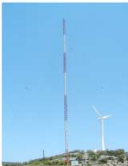
Figure 1. North-Eastwards view of the 100meter mast.
