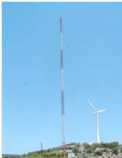
Figure 1. North-Eastwards view of the 100meter mast.
